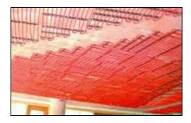
Figure 12: Ceiling cooling system.
