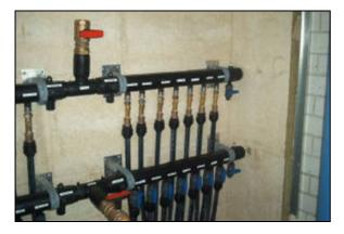
Figure 8: Manifold connecting BHEs to the heat pump(s).
