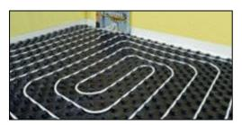
Figure 10: Floor heating system.
