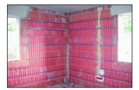
Figure 11: Wall heating/cooling system.
