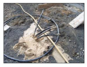
Figure 5: View of a grouted double-U BHE top
