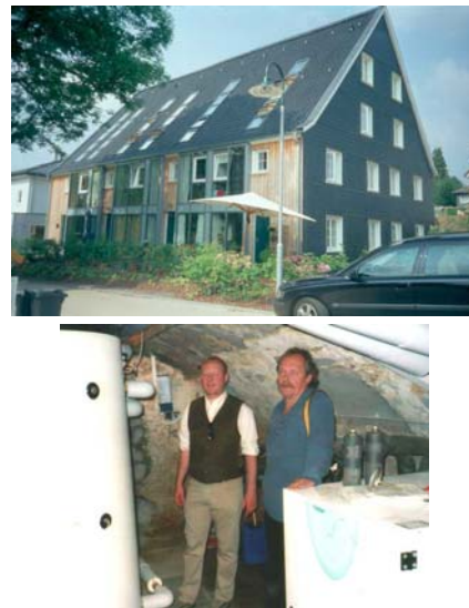
Figure 20: Hof Kolfhausen, refurbished old country mansion with GSHP and passive solar architecture; heat pump in historic vault, with GSHP-designer (left) and architect/owner (right) (photos EWS, Lund)
