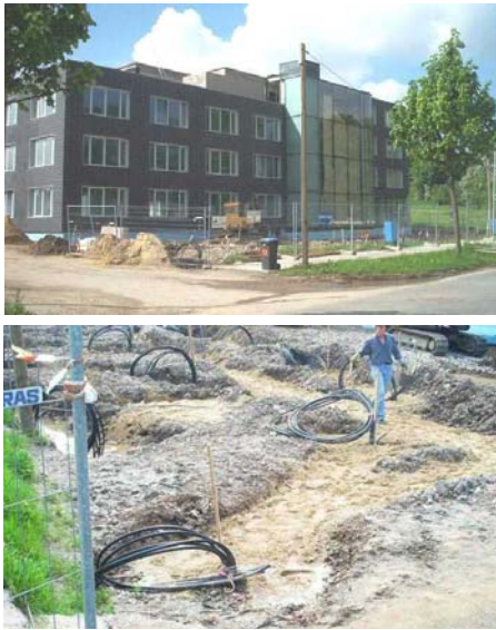
Figure 13: Office building Vika in Aachen, with the borehole field in front, and view to the BHE field with sand layer in trenches ready for receiving the connecting pipes (photo EWS)
