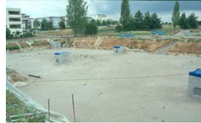
Figure 38: Plan of the store with 3 different construction stages, in 2004 final size 528 BHE (graph ITW); below 2 nd extension under construction, BHE installation completed, before top insulation (photo Sanner)
