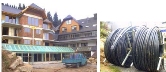
Figure 22: Annex to hotel “Schlehdorn” in Altglashütten under construction, and large reel with 250 m BHE (photos Systherma)
