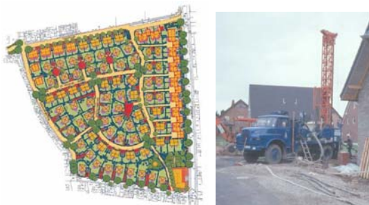
Fig 35: Plan of geothermal subdivision in Werne (each house with own BHE, graph Behr+Partner) and drilling for BHE in Werne (photo Sanner)
